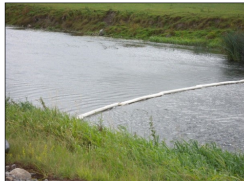
Photo 2: Installed spill boom
